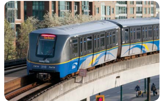
Rail Rapid Transit
